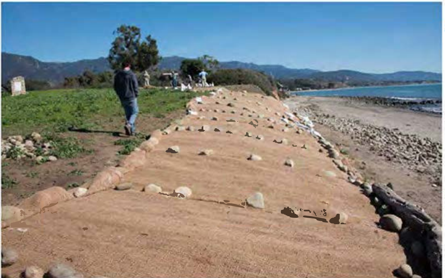
Photo 12. Erosion control being installed on bluff. February 4, 2016.
