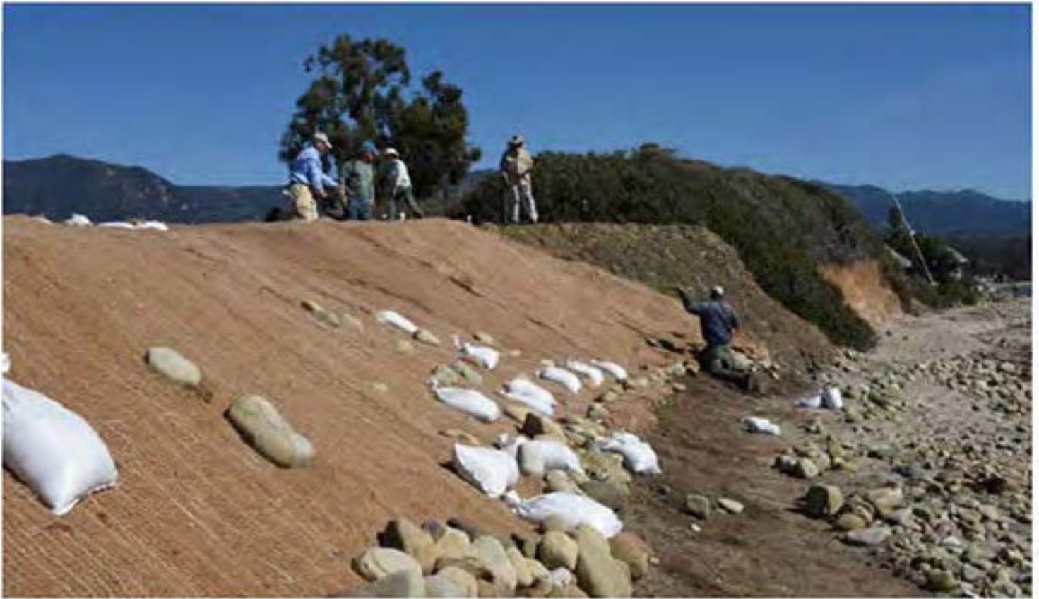
Photo 11. Erosion control being installed on bluff. February 4, 2016.
